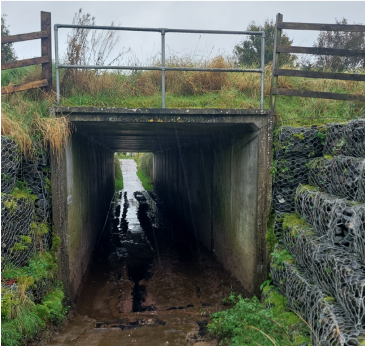
Figure 2-25: Image of Box Culvert as Cattle Underpass
