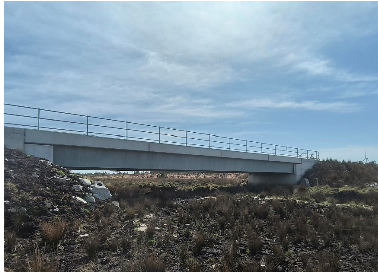
Figure 2-29: Typical Example of a Clear Span Bridge
