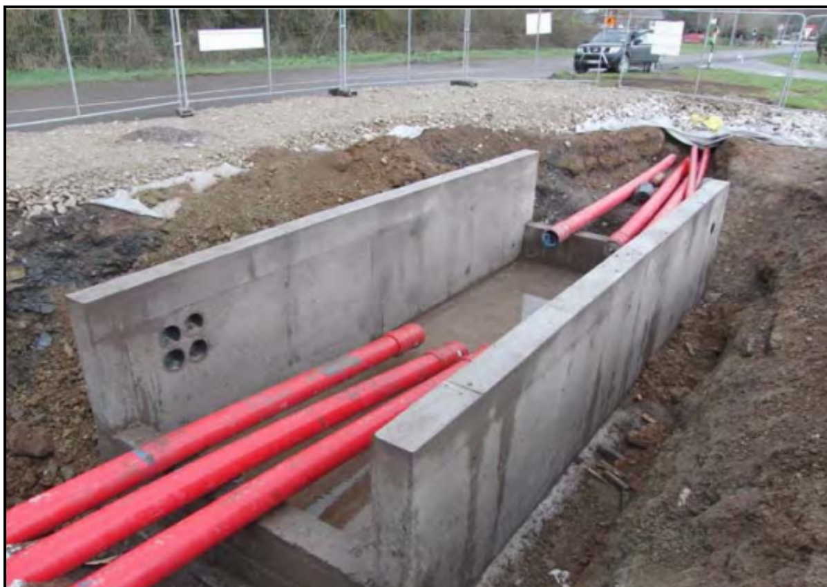
Figure 2-26: Typical Construction Process of a Joint Bay
